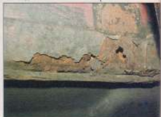
Sills are often weak, and the lower edges are especially vulnerable. If you are looking at a mixture of holes, rusty steel and various patches, bargain on extensive repairs further in!
