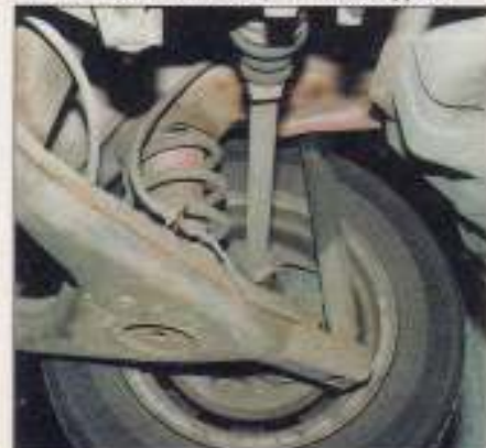
At the rear, check out the driveshaft gaiters, mounting bushes for the rear sub-frame/trailing arms, and condition of the steel suspension components. Deficiencies here spell MoT failure.
